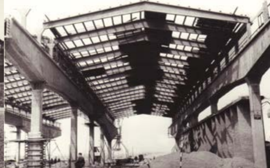
Construction of the main halls
