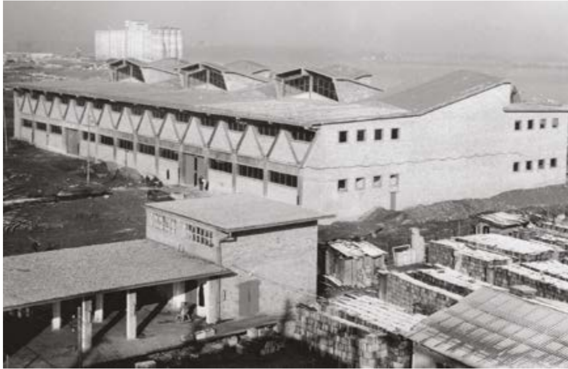
Mixed goods warehouse (1959-1961)
