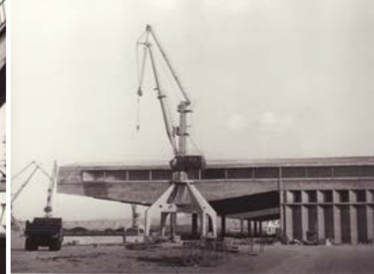
Main halls with cranes (1962-1963)
